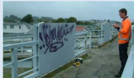
Ava on the Hutt line in Wellington suffers from graffiti attacks and was rated the lowest at 25%. The station was being repainted when photographed.
