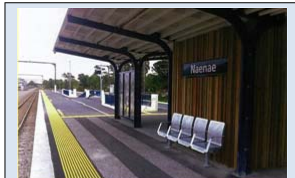
A major upgrade of Naenae station was undertaken in 2012 with the platform surface renewed and shelter replaced. The increase in passenger rating was substantial at 44% points (2003-2013).
