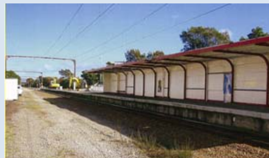
Naenae station before upgrading. (Photo provided by Steve Bird of GWRC)
